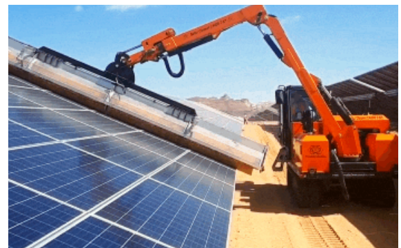
LAVAGGIO PANNELLI SOLARI SOLAR PANEL WASHING
